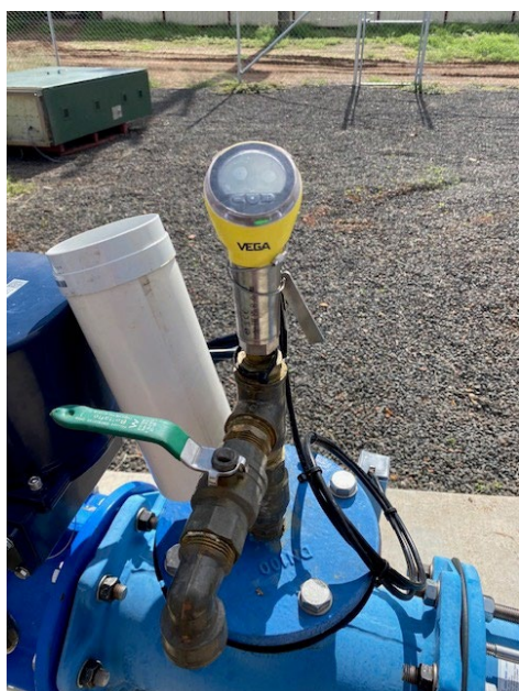
Failed Sensor on Bore 4
