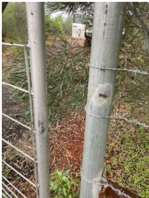
Fence and gate cut at Evaporation Ponds
